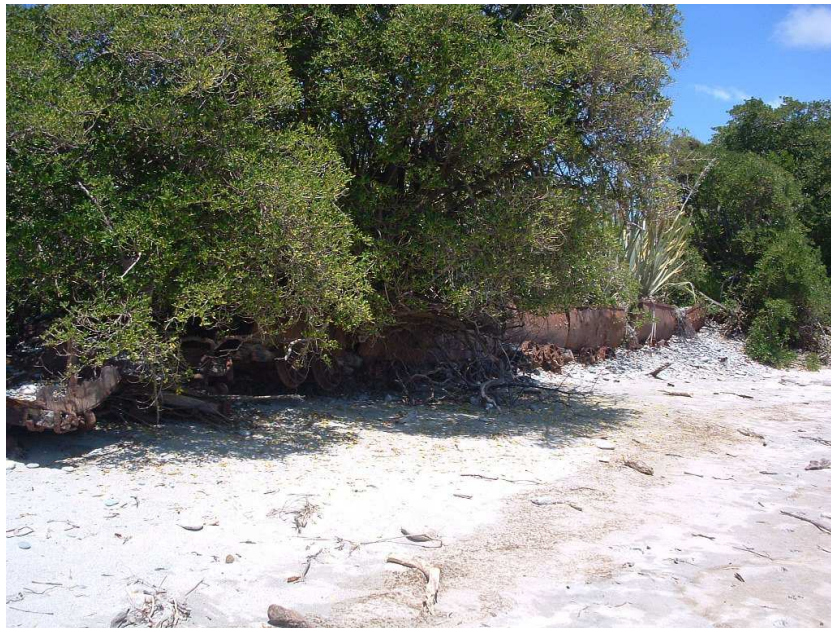
Figure 12: Old coal wagons at 31 Main Road Hector, Again these will do little to prevent ongoing erosion during storm events.
