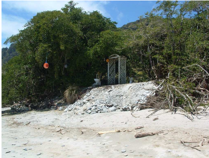
Figure 11: Rubble fill tipped over the upper beach at 29 Main Road, Hector which will be eroded away the next time waves reach the fill material.
